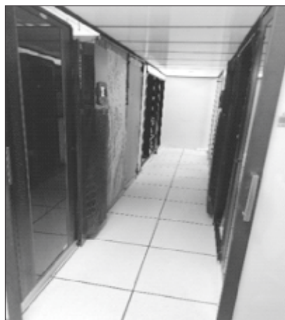
Cold Aisle Containment Passage in between Server Racks
