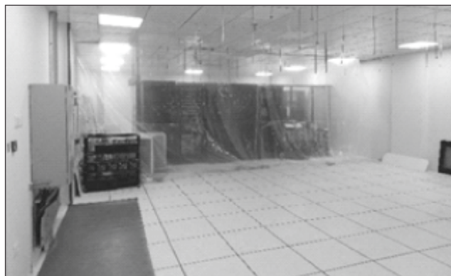
Row 1 with Cold Aisle Containment at present
