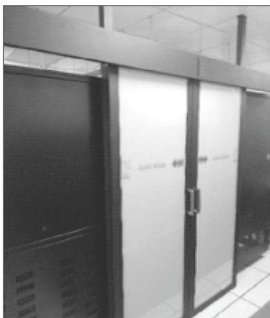
Cold Aisle Containment Entry
