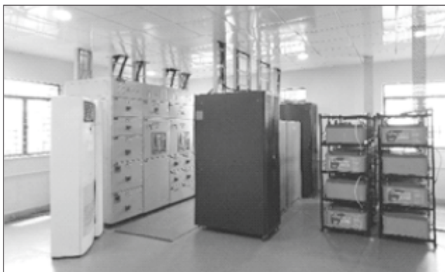
UPS along with battery bank in Electrical UPS Room
