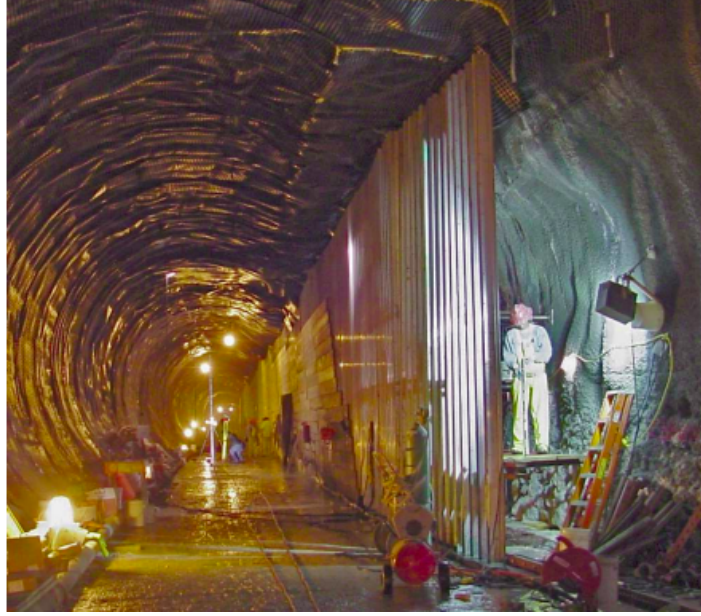
Figure 2.3: The NuMI Decay pipe tunnel before the decay pipe was installed. The wall is for the concrete shielding. The figure is taken from [10].
