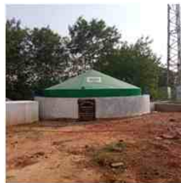
Main Digester Tank (50 Cu M)
