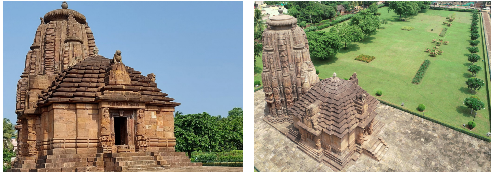
Fig. 6.6: The Rajarani Temple in Bhubaneswar, India. Left: ground-level view showing the deula (sanctuary tower) and jagamohana (porch) with intricate stone carvings. Right: aerial view showing the temple compound layout and spatial relationships between structures. The temple spans 23.7\text{m} \times 12.2\text{m} with the deula rising to 18.5\text{m} and jagamohana to 12.1\text{m} .
